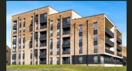
Link Housing Riverside, Dalmarnock
